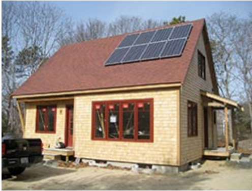
One of the new units at Jenney Way features solar panels. Click photo for larger version.
